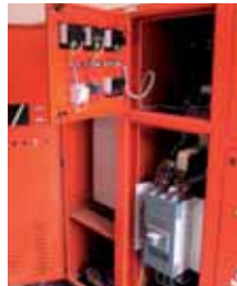
opposite page, from left: Track repair work from left: Street lighting on the CTIA approach road. On-track screener. New rail track (Exxaro project). Substation equipment installed by RACEC Electrification.
